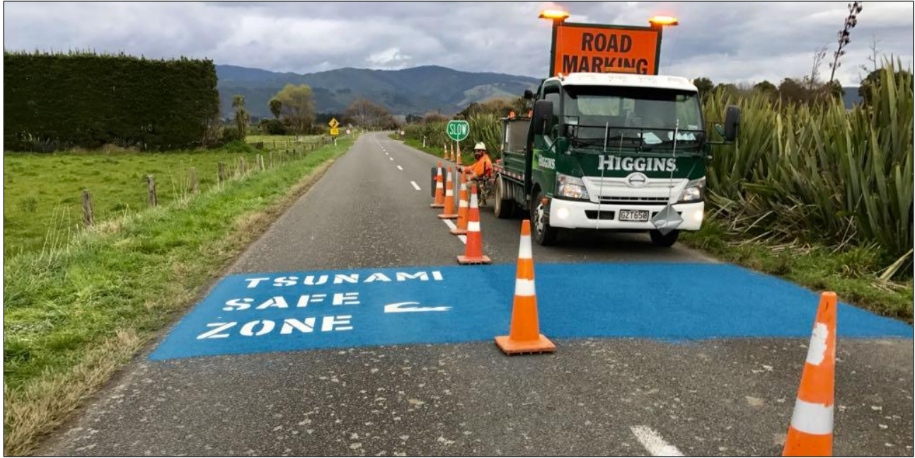
Figure 12: Example of Tsunami Safe Zone Road Marking from New Zealand (Source: Waikawa Beach Ratepayers Association )
